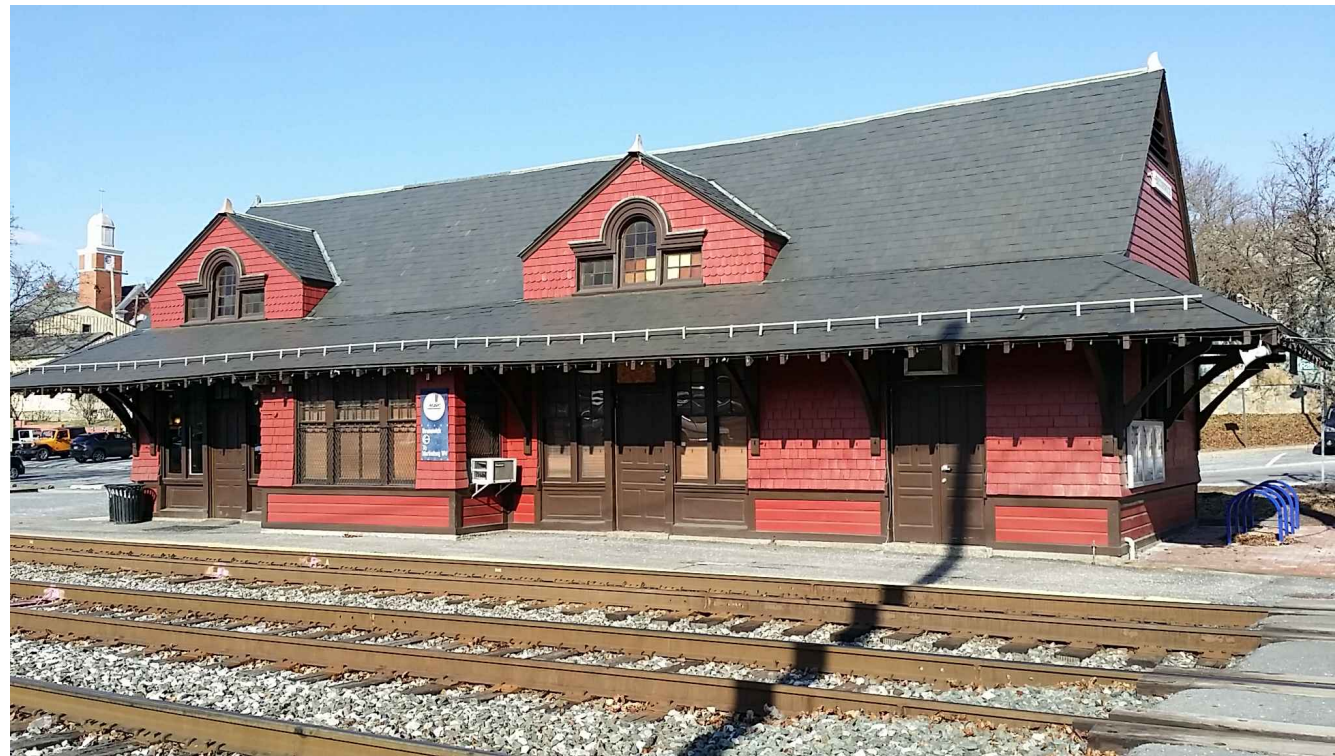
Existing Depot/Ticket Building - Looking North
